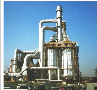
No.3 CDU, Crude Charge Heater
