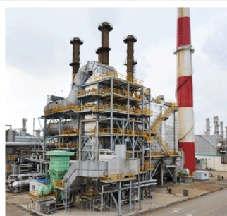
No.2 CDU Revamp Work
