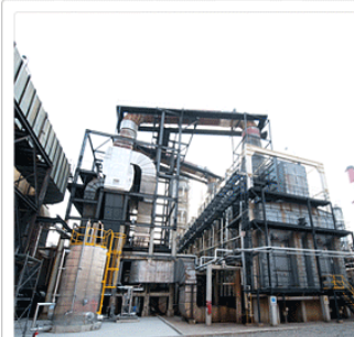
No.3 CDU Revamp work
